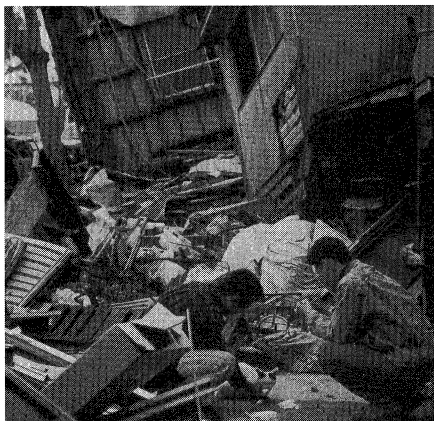
Cleaning up in the aftermath of the Great Kobe-Osaka Area Earthquake of 1995
